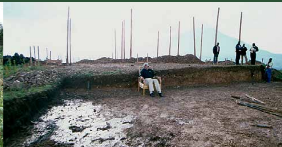
Praveen overseeing fondation work
