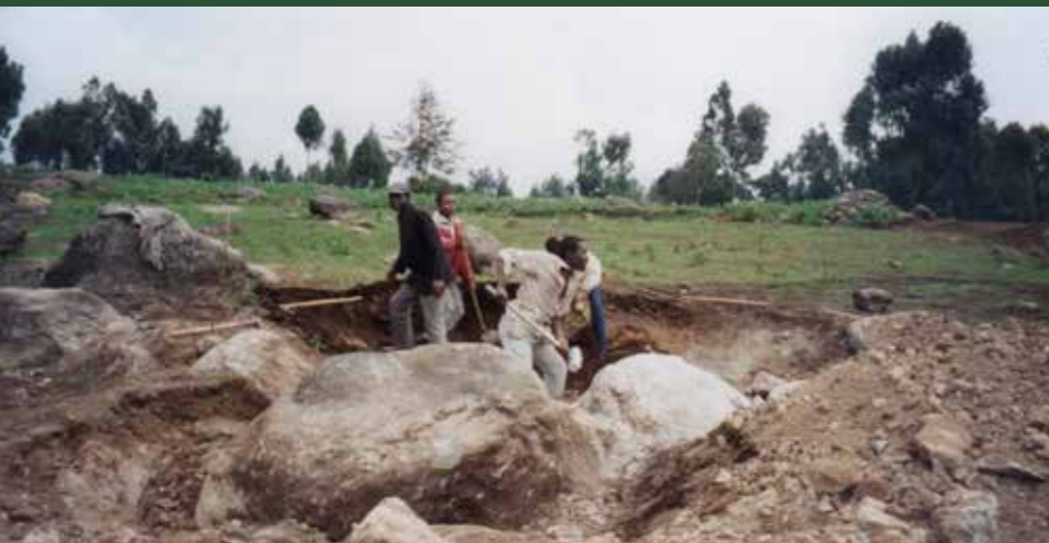
Preparing the site
