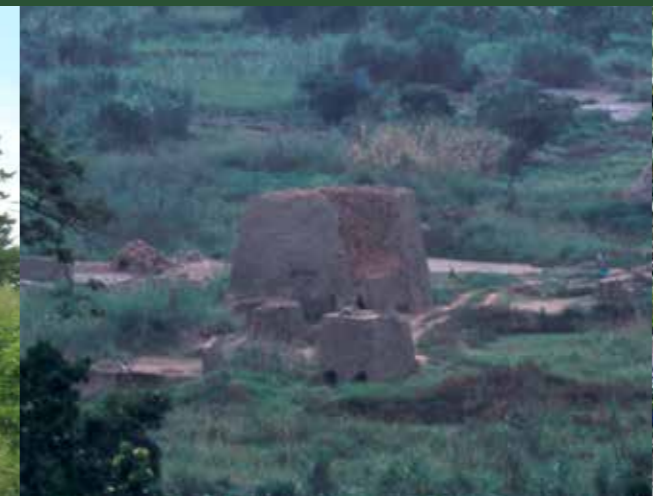
Illegal brickworks in wetland near lodge
