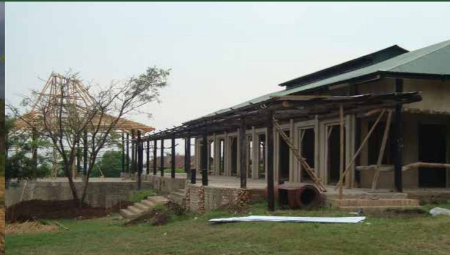
Main building remodelling
