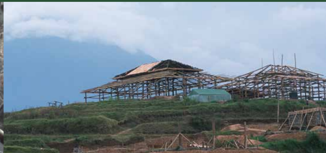
Building the public areas
