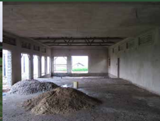
Renovating the old coffee shed
