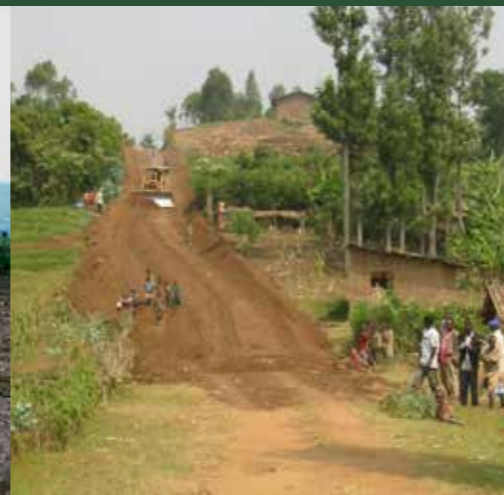
Building the 4 km road
