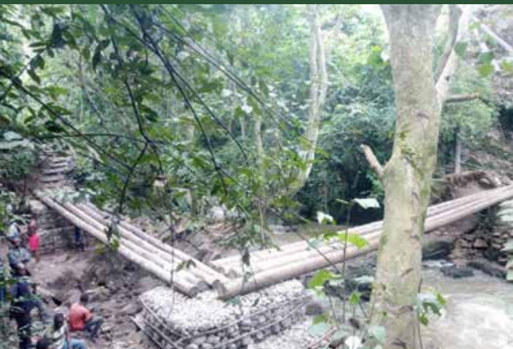
Building bridge across river
